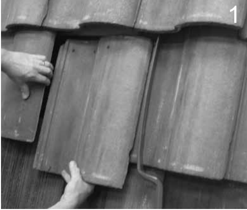
1 Remove Tile at selected location of Mount.
