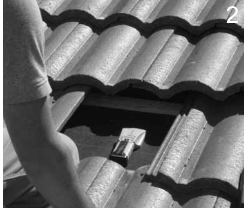
2 Locate center of rafter and Mark with a felt pen.
